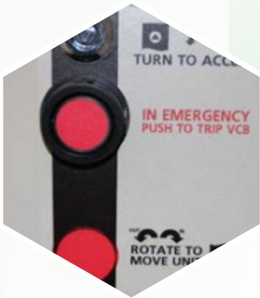
**An emergency trip push-button** is located in the center of the panel. It has a striking, protruding design protected against accidental operation. The trip button can be quickly spotted in an emergency.
